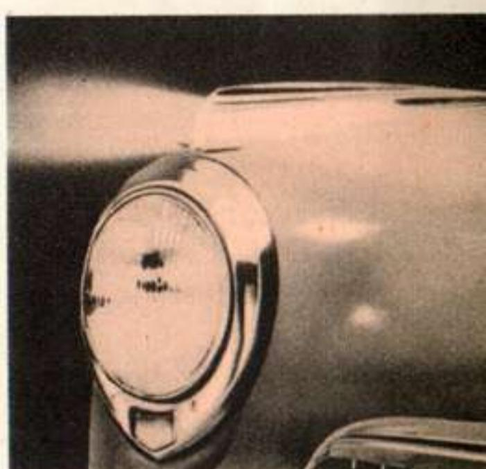
**Built-in Directional Signaling Equipment** provides convenient lever at your finger tips on left side of steering column with which to signal turns to following and approaching traffic. Special bulbs in fender and tail lamps flash brilliant warning signal. Signal turns off automatically.
