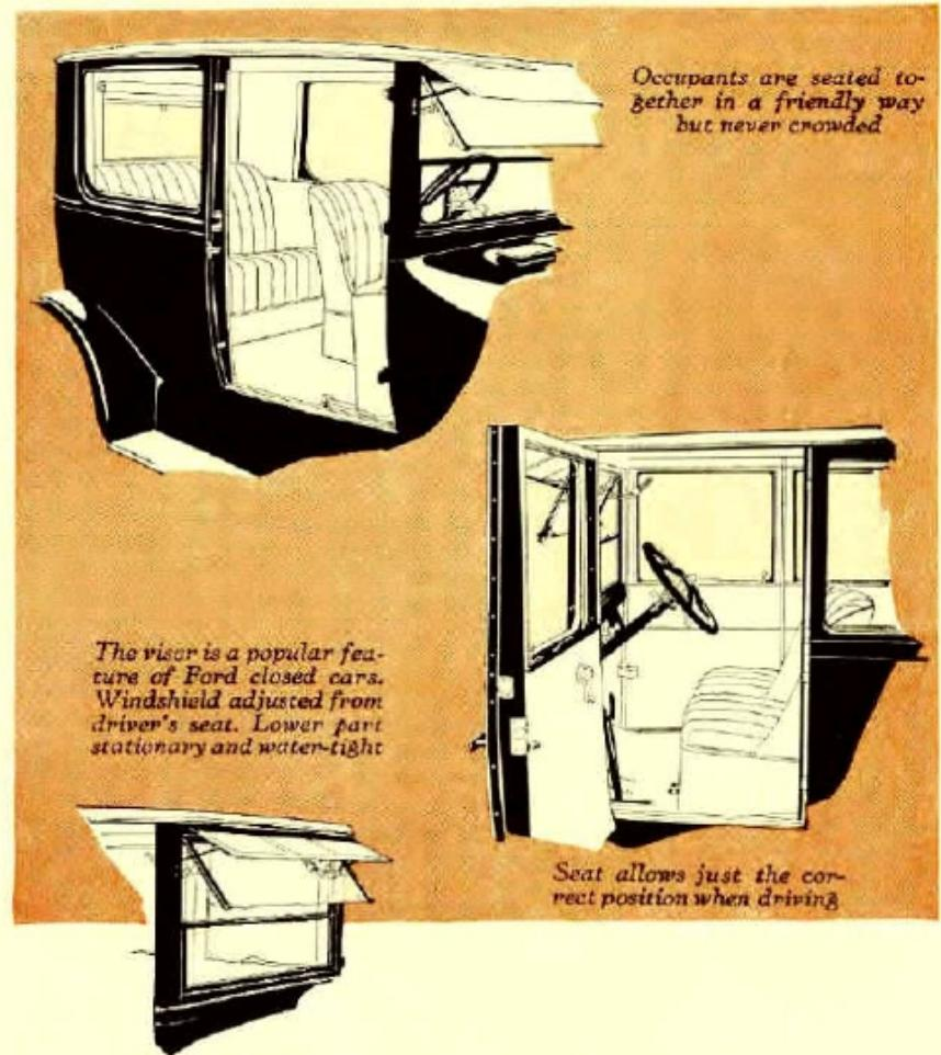
*The visor is a popular feature of Ford closed cars. Windshield adjusted from driver's seat. Lower part stationary and water-tight*
