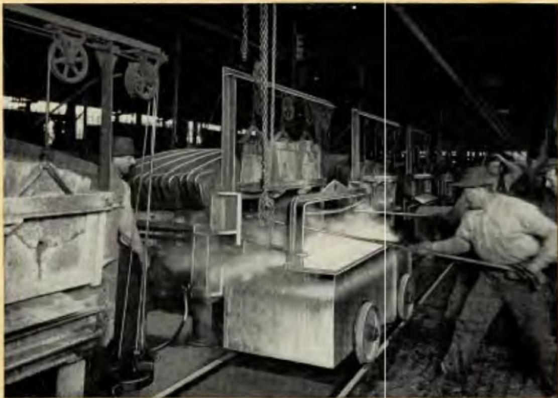
Quenching Steel Forgings in Heat-Treatment
