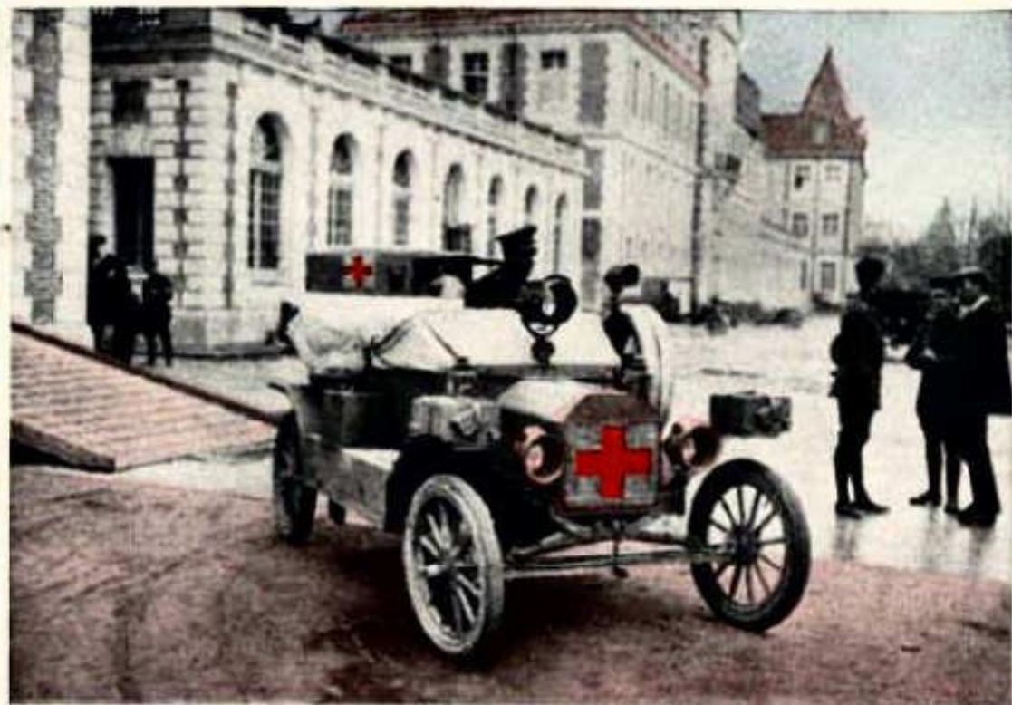
Section Commander's car. Note big tool boxes, reserve gasoline on fenders, big headlight and waterproof cover on tonneau
