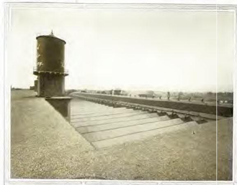
SOME ROOF —The glass saw tooth roof is over the machine shop; the crane way at the right
