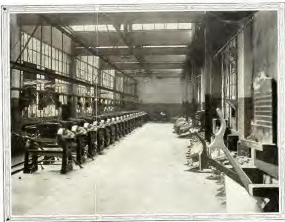
ASSEMBLING AND TESTING Ford motors. The most important unit of the car, they are put together as carefully and perfectly as a watch
