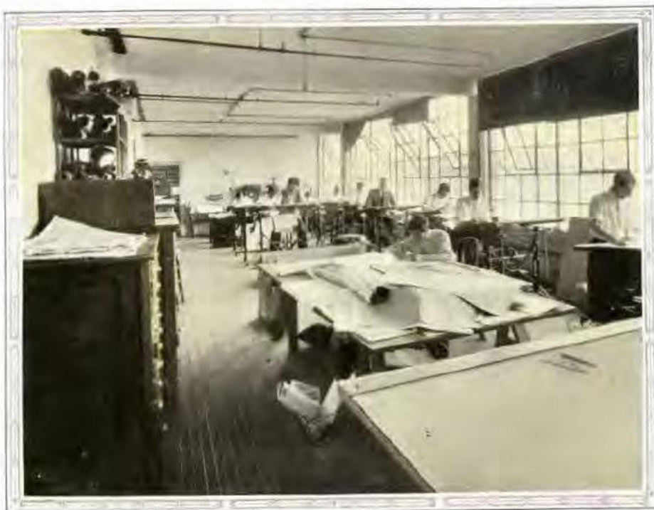
TOOL DRAFTING ROOM —Devoted solely to designing, and furnishing plans and specifications for special Ford tools and machinery
