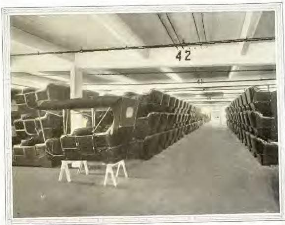
A THOUSAND Ford bodies, formed out of pressed sheet steel. It looks like a year's supply but they will all be used up in three days
