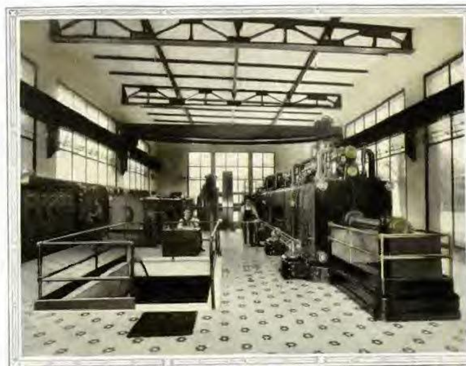
ENGINE ROOM —At the right is the great engine, then its 40 ton flywheel, the generator, air compressor and the switchboard
