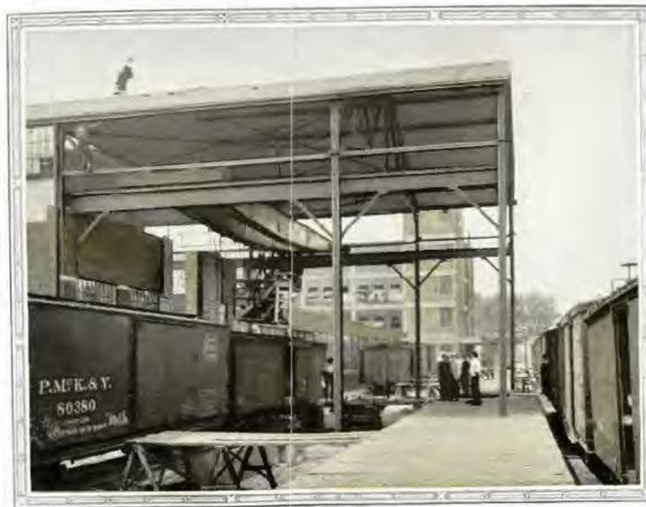
CRANE AT WORK —The ponderous screw machine suspended above the cars, weighs two tons. The crane has just raised it from the platform
