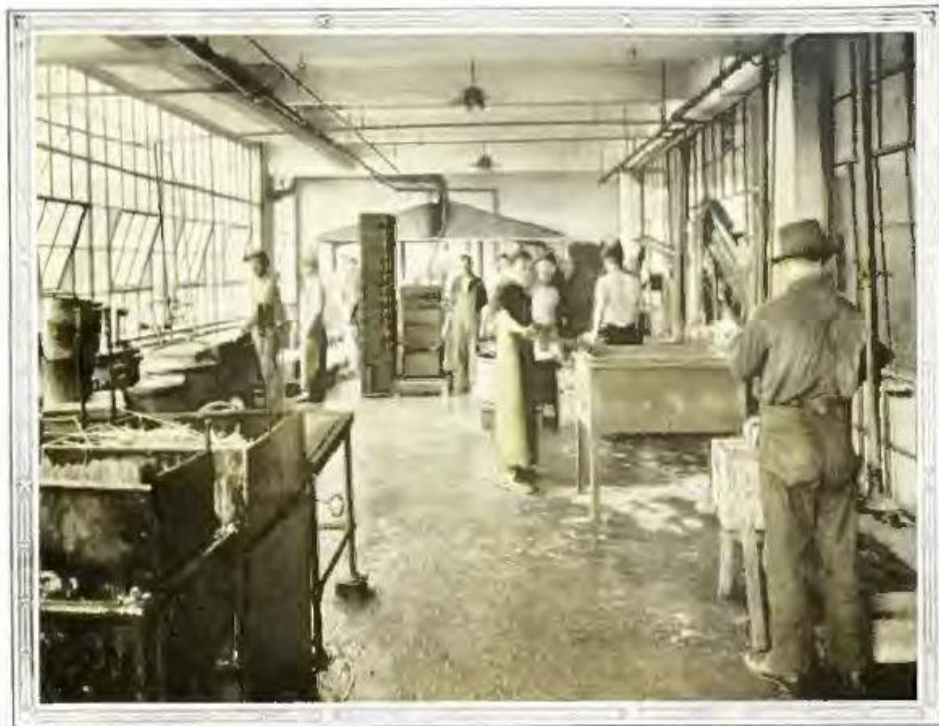
TINNING RADIATOR PARTS —Making them rust proof, leak proof and generally dependable for a long term of years
