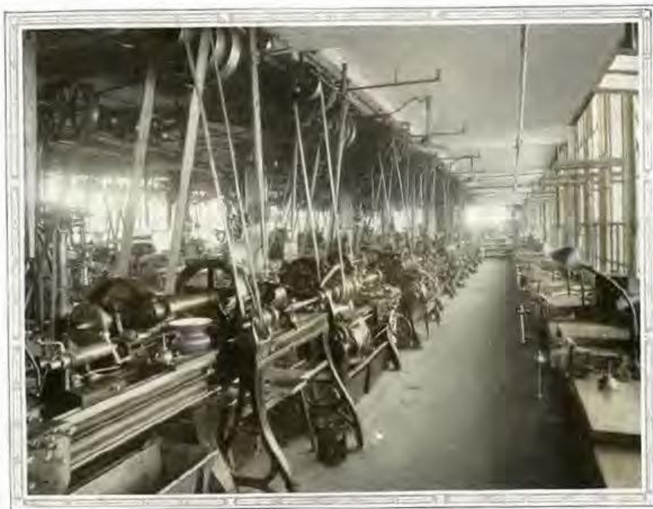
TOOL ROOM —This big shop is employed solely in making tools, jigs, dies and special parts for the mammoth machine shop
