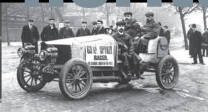
1903, SPYKER 60 HP, THE WORLD'S FIRST SIX-CYLINDER FOUR-WHEEL DRIVE CAR
